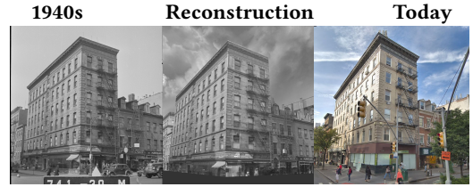
(a) 7th Ave, 17th St, NW Corner.
